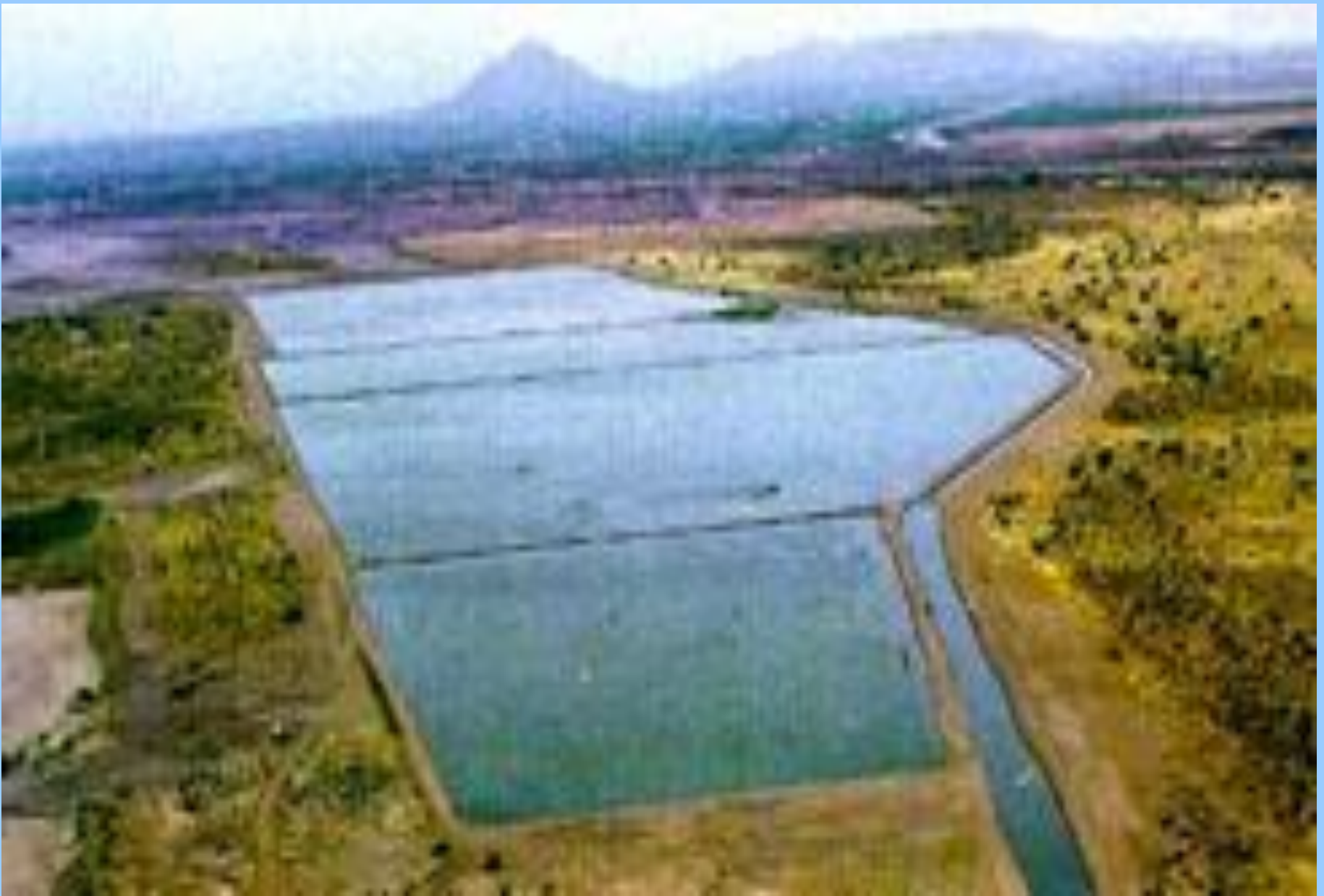
Granite Reef Underground Storage Project Recharge Basins
